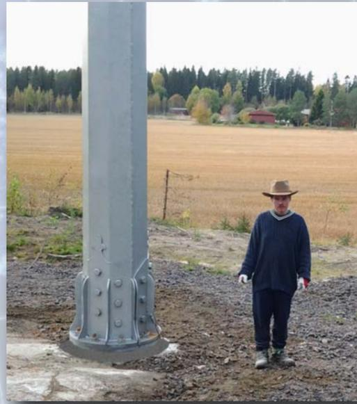
The cell structure of the mast combined with high tension steel makes the weight of tower to be only one third of what it is with traditional tube masts. The tower is probably the most light-weight and still the strongest self supporting tube mast available. Just think about the raw material saved.
