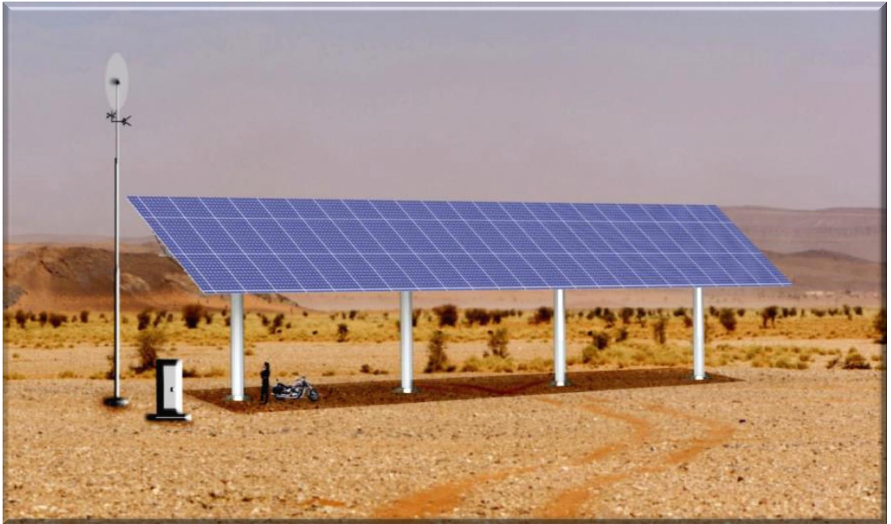
Quattro Solar Energy Tower in vertical sun tracking -100 kW (Without horizontal turning)
